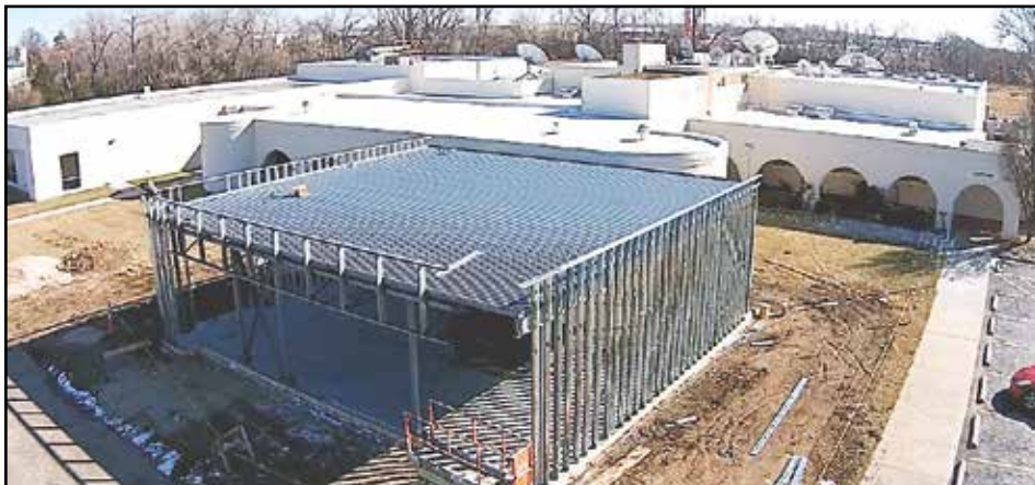
Addition to the Sunflower Broadcasting complex under construction
